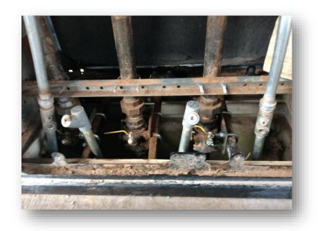
This picture is taken from underneath a dispenser. The presence of ball valves (see yellow handles), underneath breakaway valves, invalidates the breakaway valves. The ball valves need to be replaced with a proper plug from the respective manufacturer. This is a safety issue.
